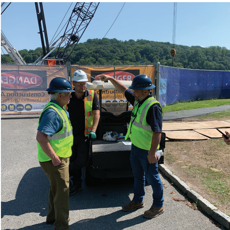
Assemblymember Lavine toured the construction site of a major engineering project at Cold Spring Harbor Lab. The Lab's mission is to shape contemporary biomedical research and education with programs in cancer, neuroscience, plant biology and quantitative biology. Lavine helped secure funding for this, and other projects, at the lab.
